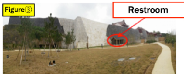
Image of the Northern Castle Wall East Area after the improvement construction
