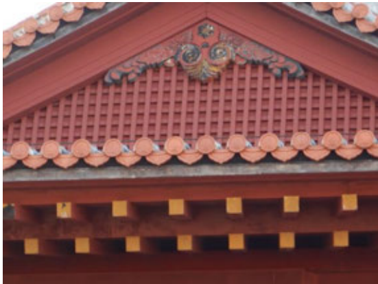
【Gabled section: Gegyo (decoration board), rafters, etc. -- colors have faded】
