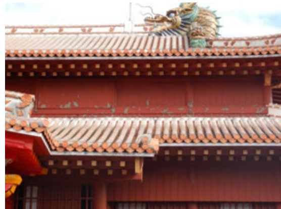
【Outer wall section - the lacquer has peeled off】
